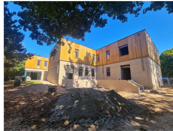
Dartmouth Health Hub: image extracted from August 2022 Contractor Report
